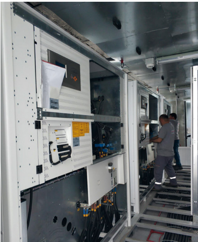
3x600kVA Parallel Containerized Shore Power Converter with HVAC, Control Panels and Communication options.
